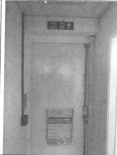
10- Unit 11 fire exit route to rear
